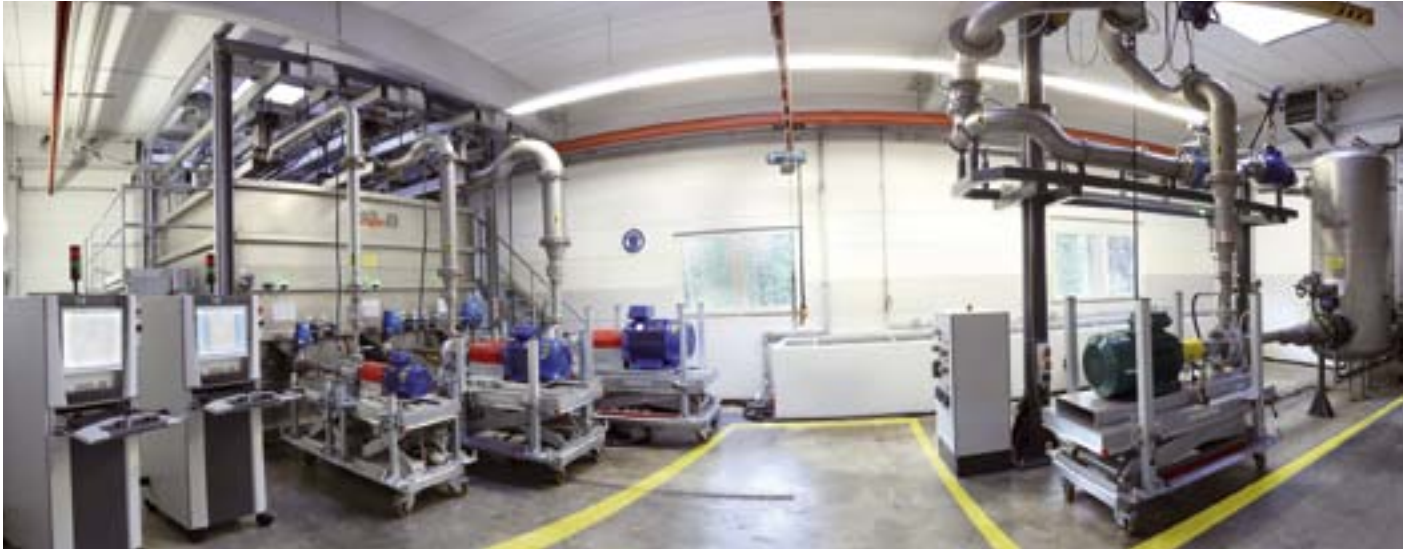
Computer-controlled and fully automated test stands on the premises of Speck Pumpen in Roth. Measuring of hydraulics, power requirements, axial thrust, vibrations and NPSH values. Heads of up to 400 m and flow rates of up to 750 m 3 /h are possible.
